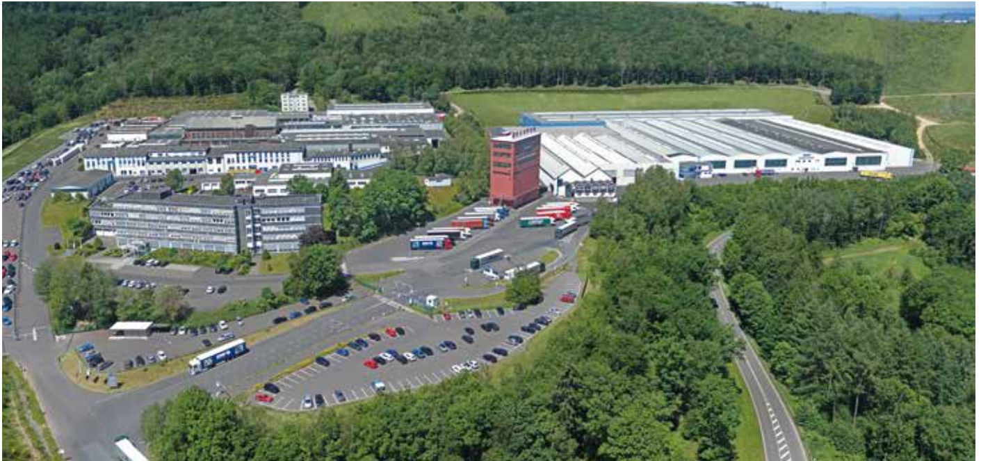
Head office and plant, Neunkirchen, Germany
